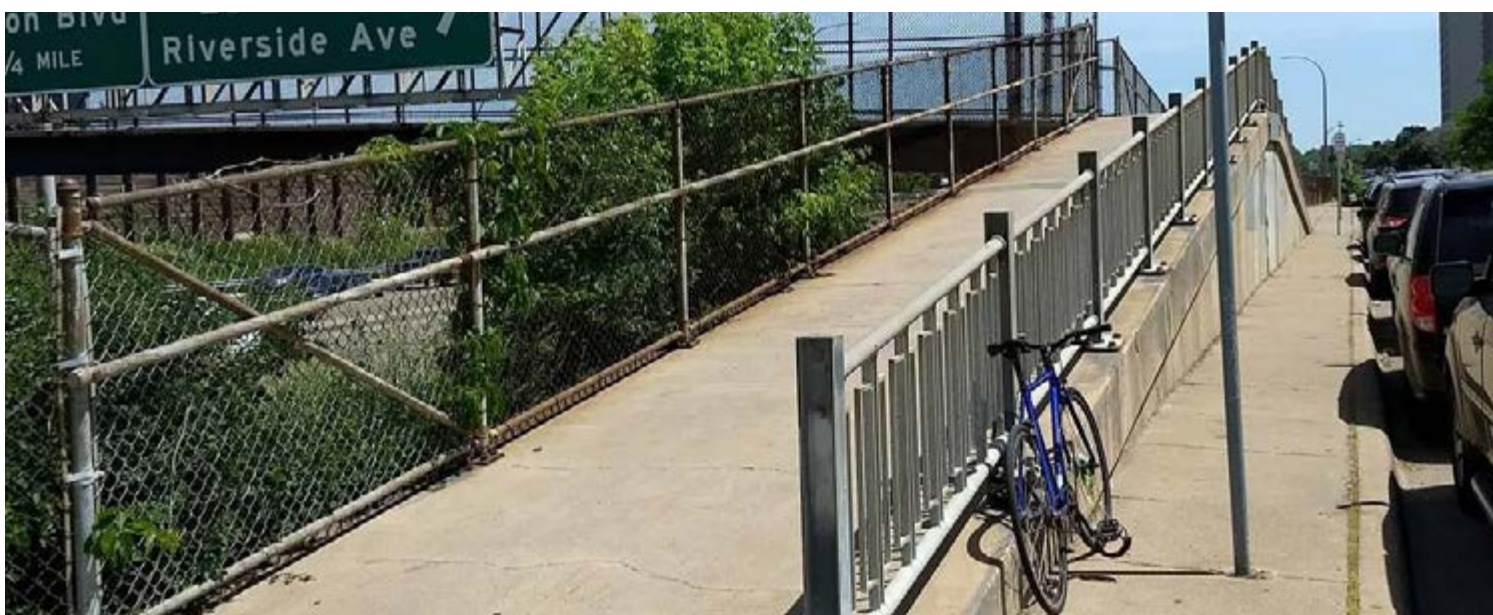
Figure 5 Non ADA compliant ramp system on South end
