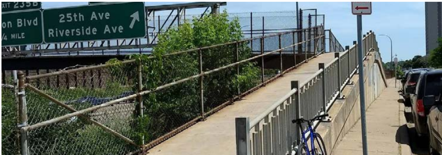
Figure 3 Limited visibility and steep ramps at Murphy Park Pedestrian Bridge
