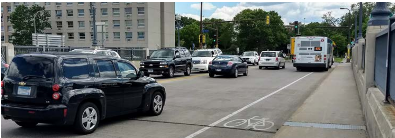
Figure 4 Narrow sidewalks and bike lanes adjacent to traffic on 25th Avenue bridge
