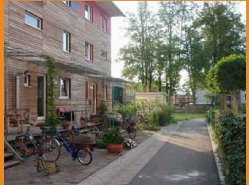
Example of variety of functions at parcel edges, Freiburg, Germany.
