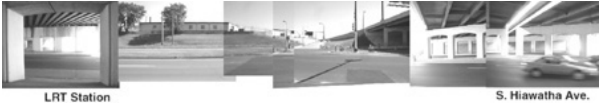
Figure #10: South side of Franklin between the LRT bridge and station and Hiawatha Ave.
