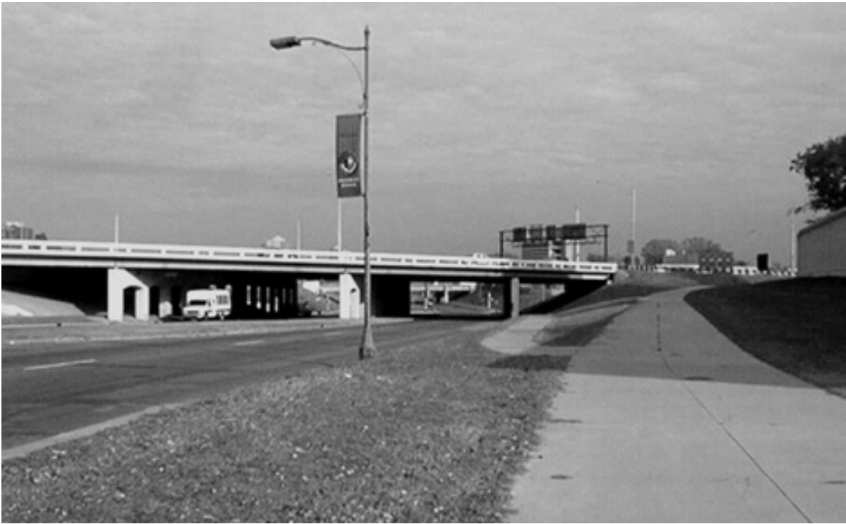
Figure #4: View approaching the LRT station area from the Phillips neighborhood.
