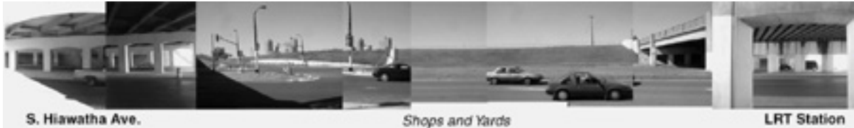
Figure #7: North side of Franklin between Hiawatha and the LRT bridge and station.
