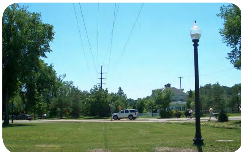
Powerline transitions from double row of Trellis Towers to Monopoles at Minnehaha Park
