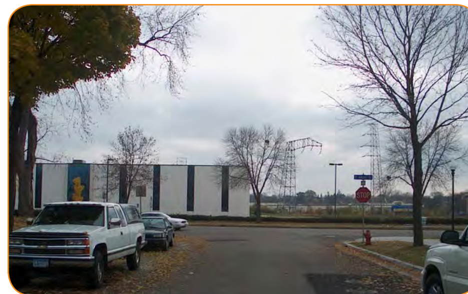
Town Square site looking south along Snelling Avenue
