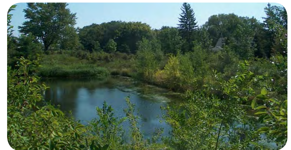
Stormwater retention pond across 46th Street from the LRT Station
