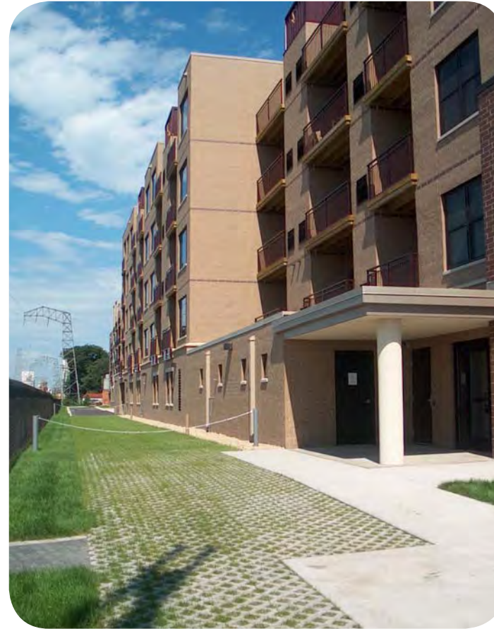
Permeable pavers that provide growing space for grass improve stormwater infiltration at Hiawatha Flats
