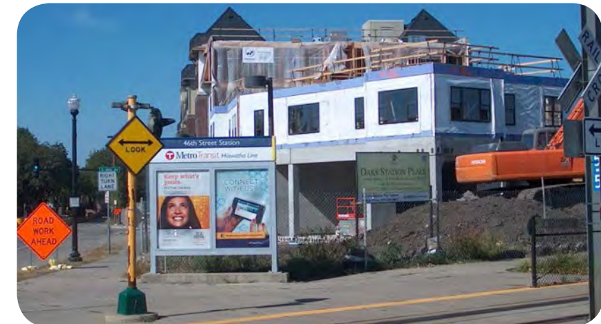
Oaks Station Place under construction summer 2012
