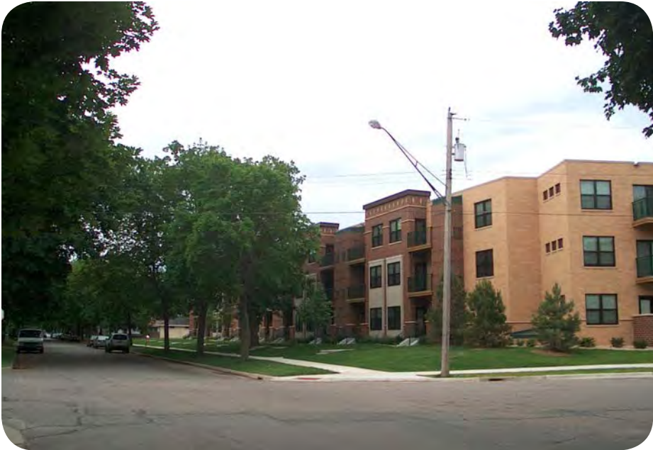
After: New Hiawatha Flats Apartments from the corner of Snelling Avenue and 43rd Street
