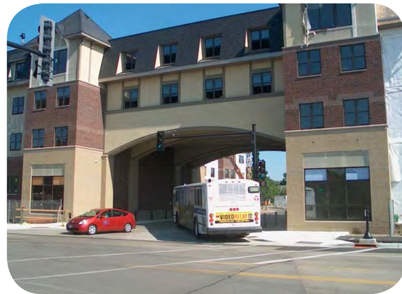
The Oaks Station Place development provides a distinctive new entrance to the transit station
