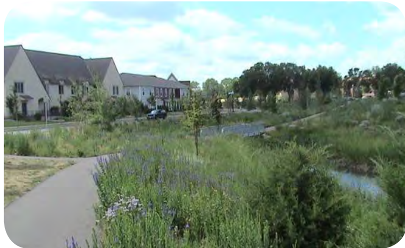
Linear stormwater infiltration facility and trail in North Minneapolis
