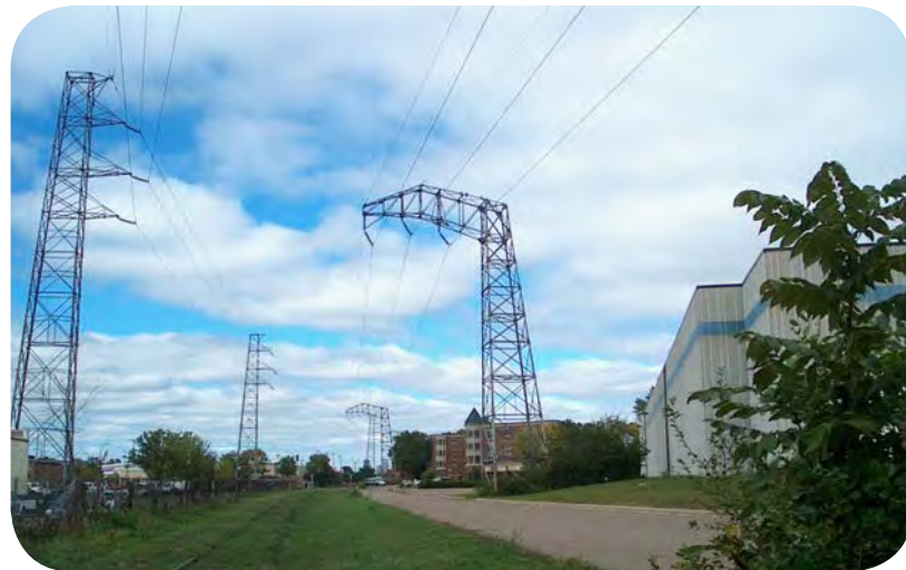
High Voltage Powerline
