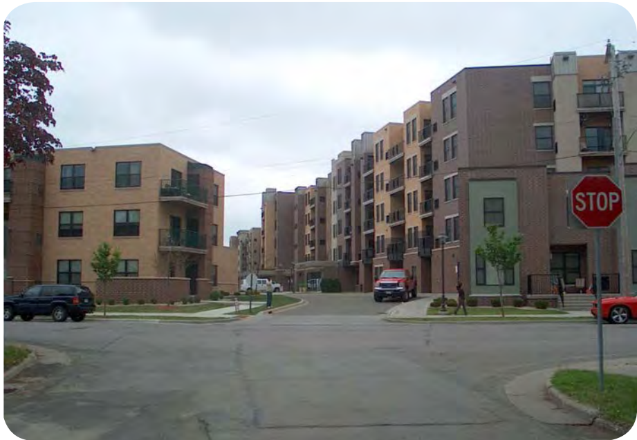
After: New Hiawatha Flats Apartments from the corner of Dight Avenue and 43rd Street
