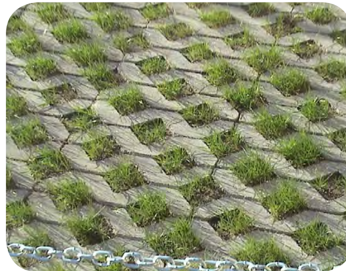
Permeable pavers that provide growing space for grass improve stormwater infiltration at Hiawatha Flats
