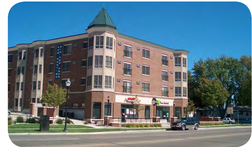
Oaks Hiawatha Station Apartments
