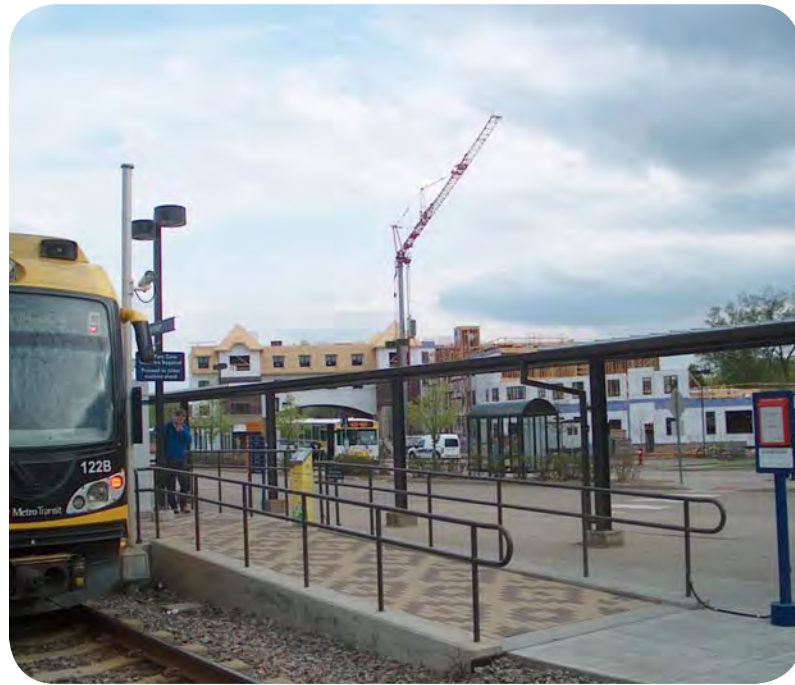
Oaks Station Place Apartments is currently under construction at the 46th Street LRT Station
