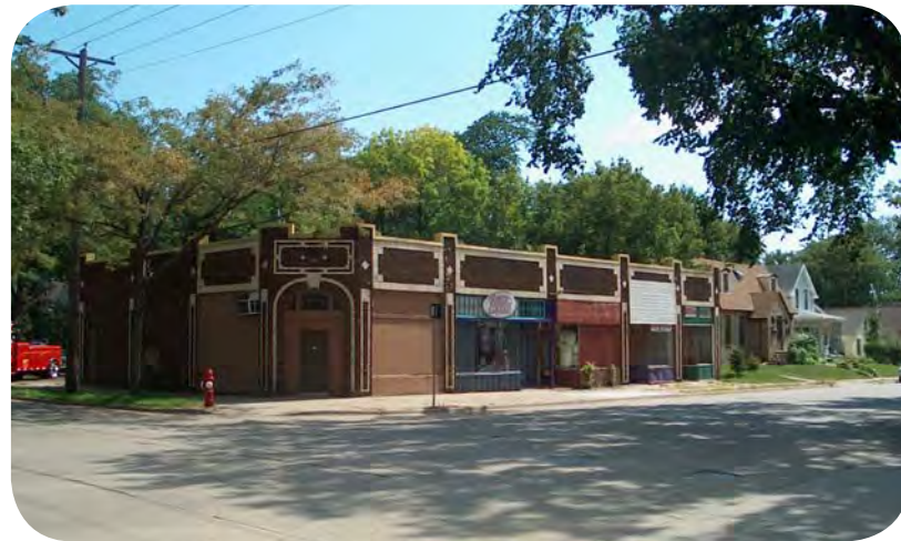
Preservation Area: Traditional Neighborhood Storefronts outside the change area
