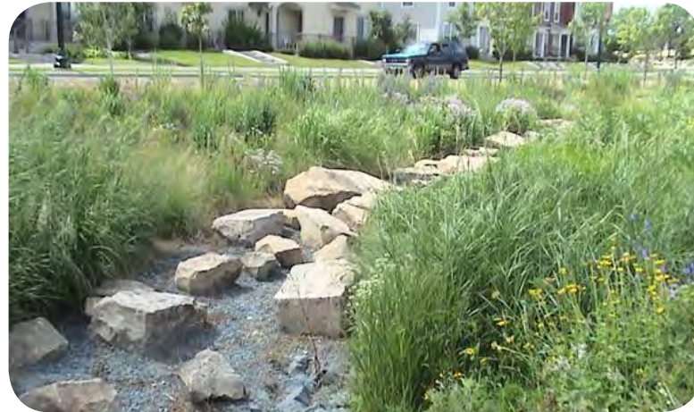
Linear Infiltration Features at Heritage Park in North Minneapolis
