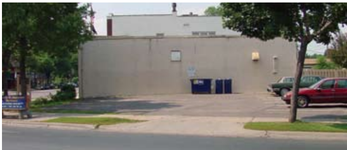
Current conditions at corner.
