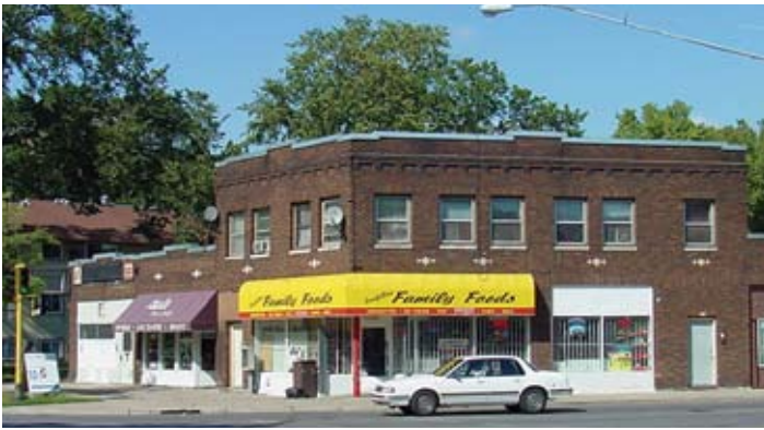
Typical one to two-story commercial building on Minnehaha Ave. & 35th St.
