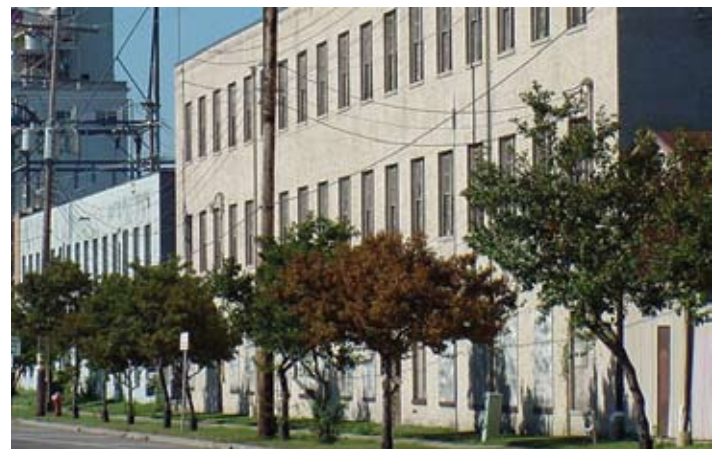
Buildings on Hiawatha with adaptive re-use potential for office, housing or light industrial.
