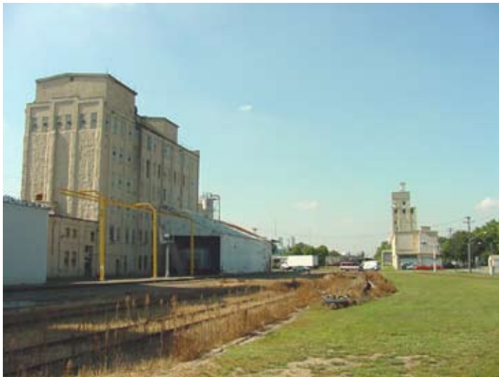
Despite their location in a industrial district, the plan supports re-use of the Nokomis and Dana Mills for office or residential.
