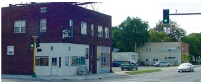
Southside of 38th St. between 27th & 28th Avenues.
