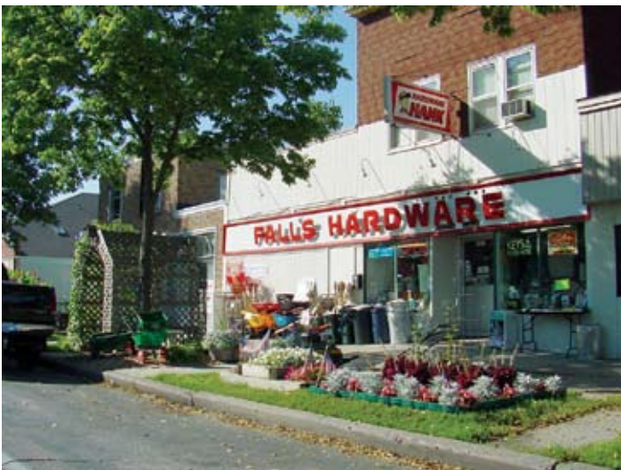
Falls Hardware at the SW corner is more consistent with the preferred character of the node than the building at the NE corner.
