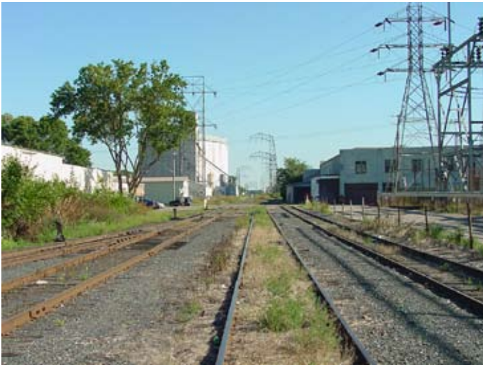
Looking south down rail corridor from 39th St.
