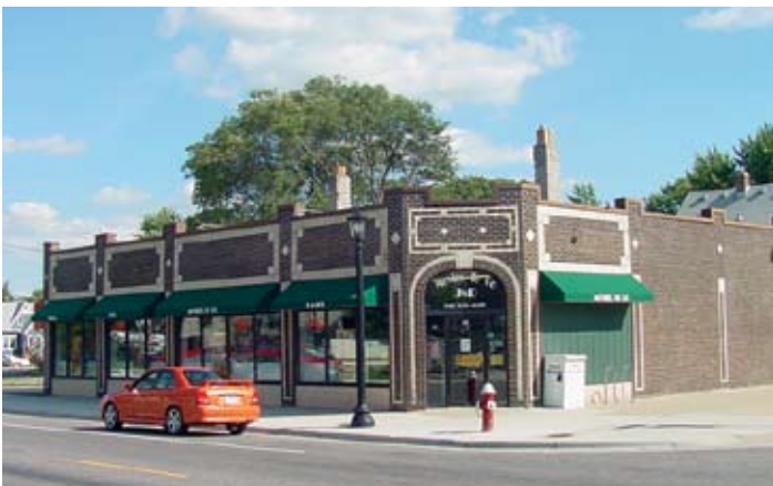
Existing commercial buildings at 38th Street & 23rd Avenue.
