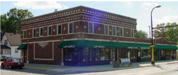
The “Bear Hawk” building at SW corner of 38th St. & 23rd Ave.
